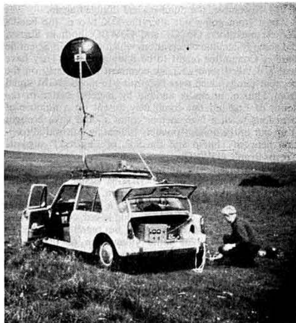
One end of the 13cm link established during the recent tests on the 2300 MHz band between G3BNL/M in the Cotswolds with G3EEZ/P who was 52 miles away near Wolverhampton. Les Sharrock, G3BNL, by starboard tail light. The 70cm aeriels used for the essential talk-link may be seen just below the 13cm dish. Subsequently signals were lifted over an 80 mile path. The tests are planned to continue when "portable" weather returns next year.
